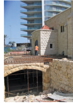
Work on the hall at All Saints'
